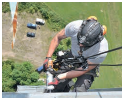
The DA1 used in windturbine assembly
